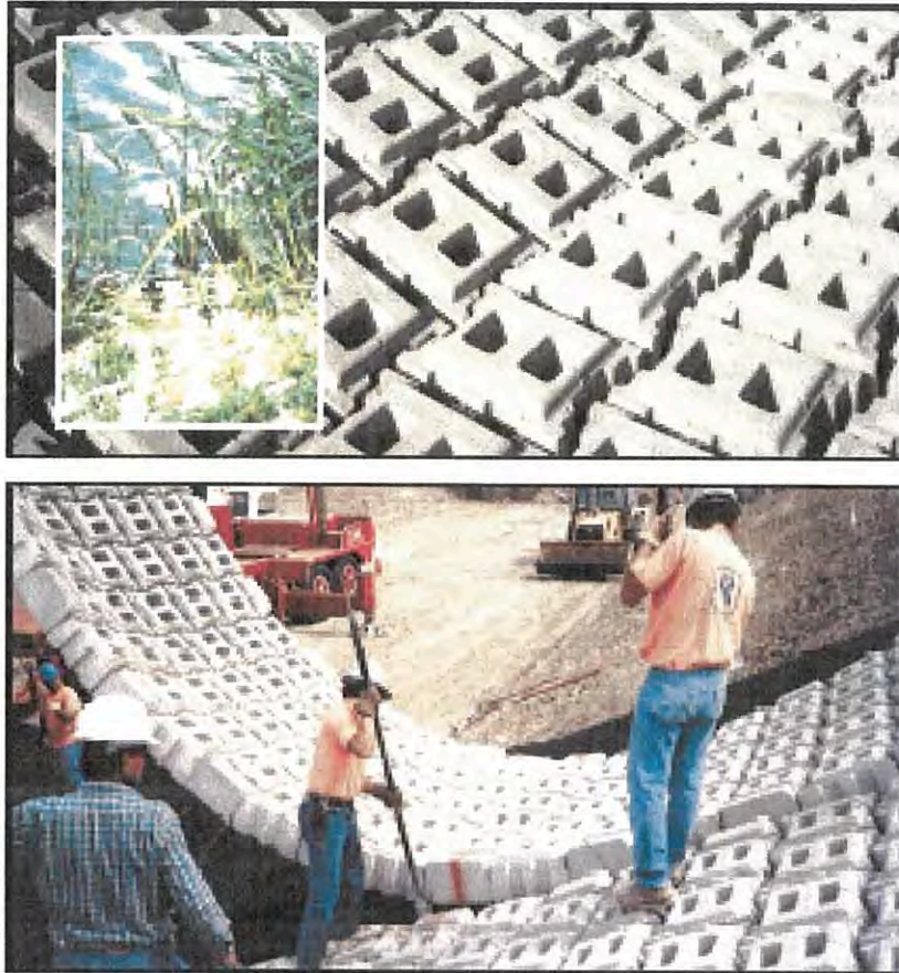
Figure 8 - Articulated Concrete Block mattress installation, close-up details, and finished appearance
