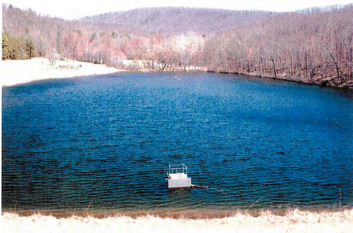
Figure 3 - Inch Branch (#26) riser and reservoir.
