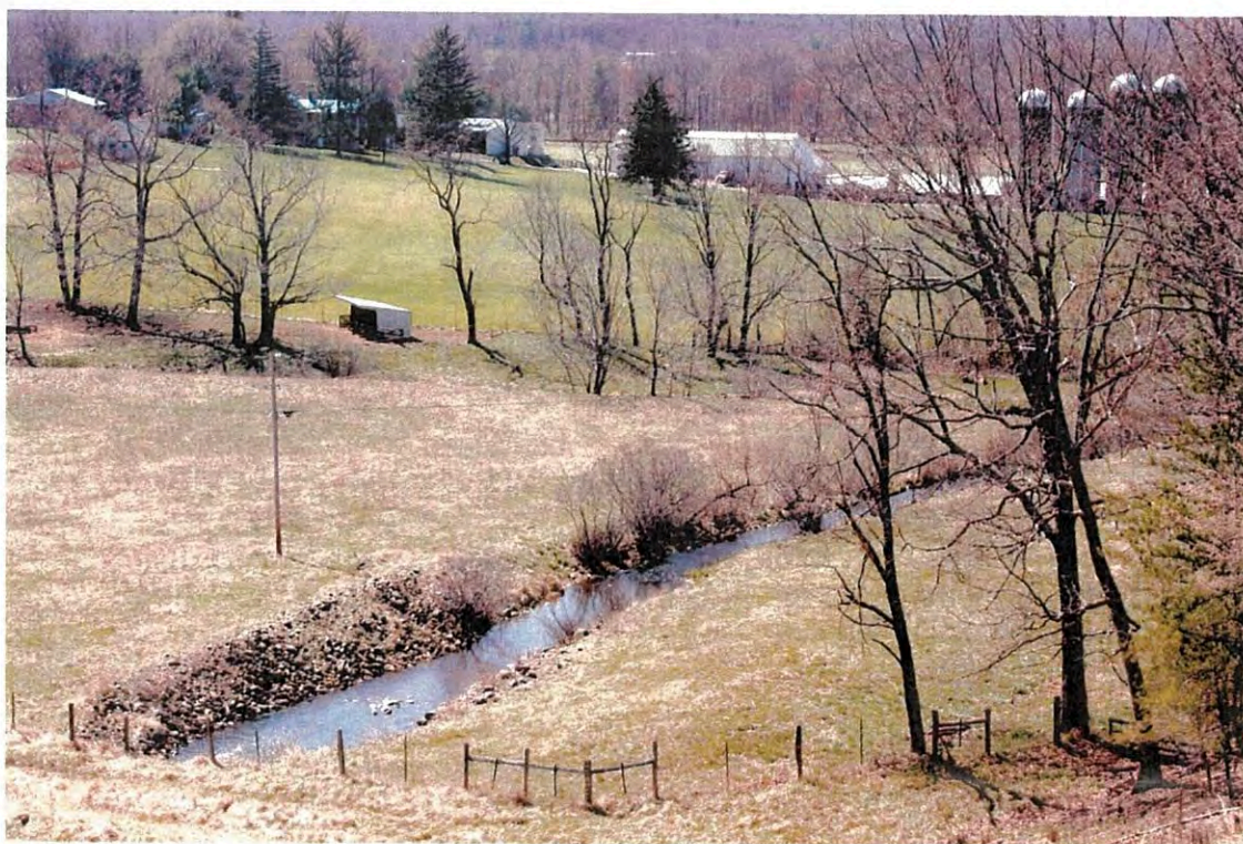
Figure 5 - Looking downstream of Toms Branch dam.
