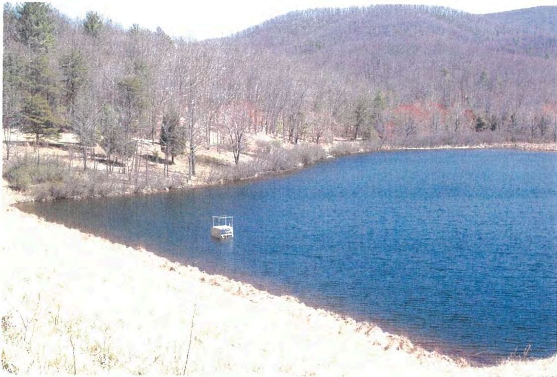
Figure 2 - Robinson Hollow (#23) dam and riser.
