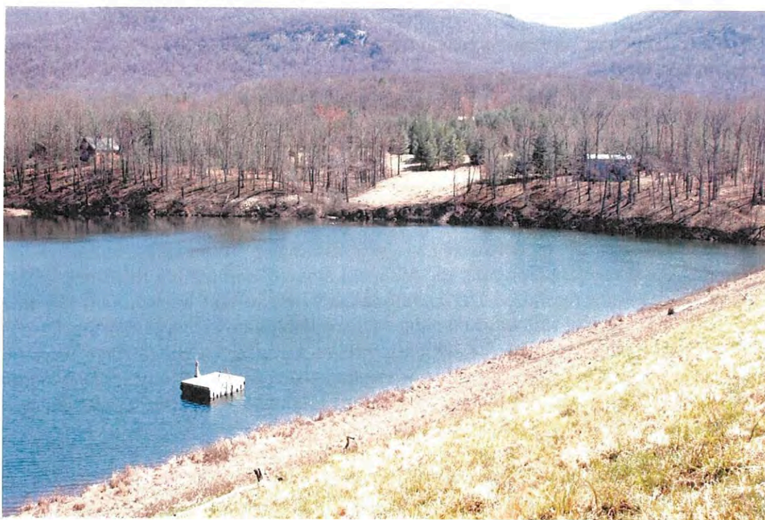
Figure 4 - Toms Branch (#25) dam, looking upstream at the riser and auxiliary spillway.
