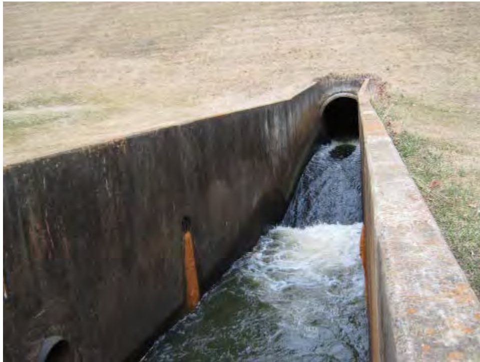
Figure 2. Principal spillway outlet pipe, chute spillway, and drains below dam.
