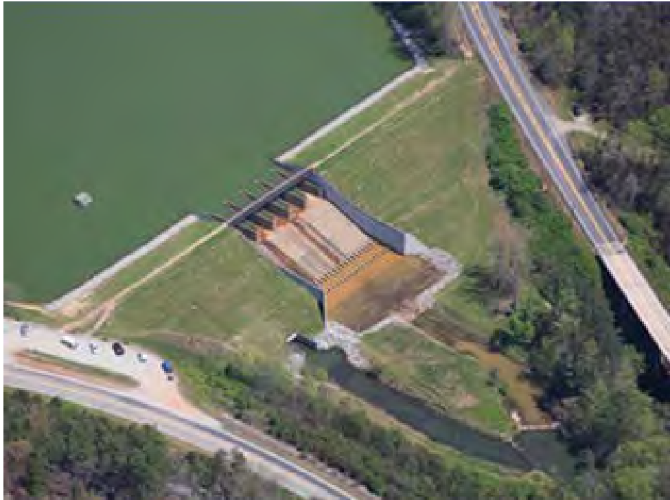
Figure 7. Example of a 5-cycle labyrinth weir.
