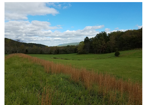
Vegetated earth auxiliary spillway
