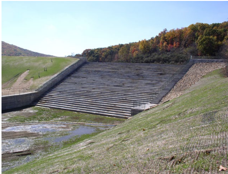
Figure 3. Example of an RCC auxiliary spillway over top of a dam.
