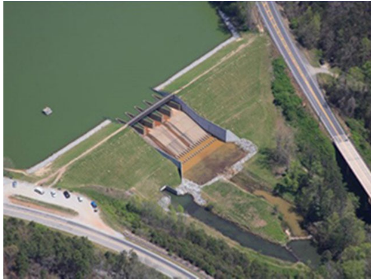
Figure 2. Example of a labyrinth weir auxiliary spillway with five cycles.
