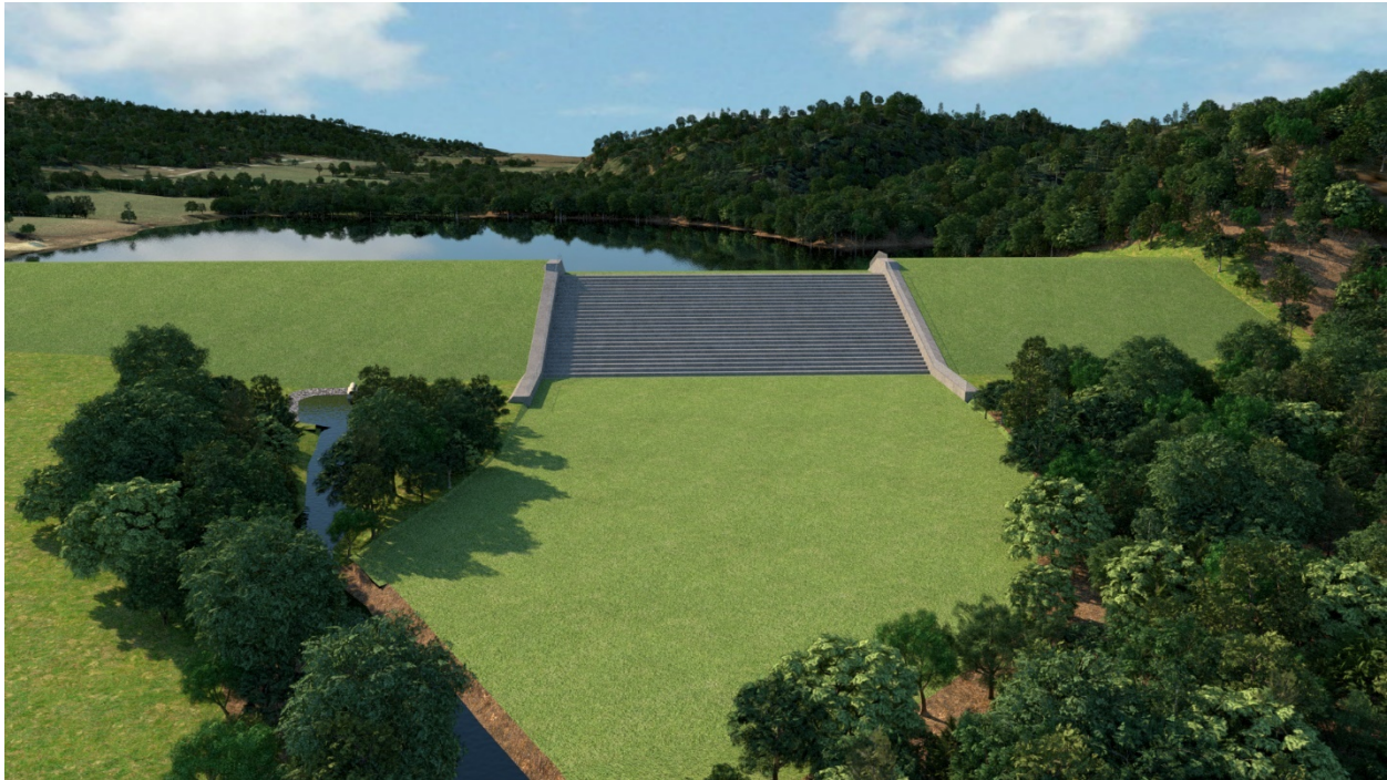
Figure 7. Rendering of the 270-foot-wide RCC chute spillway looking upstream at the dam.
