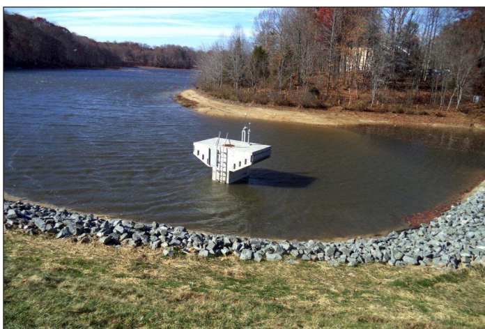
The open spillway riser (above) was replaced to improve public safety and prevent clogging from floating debris.
