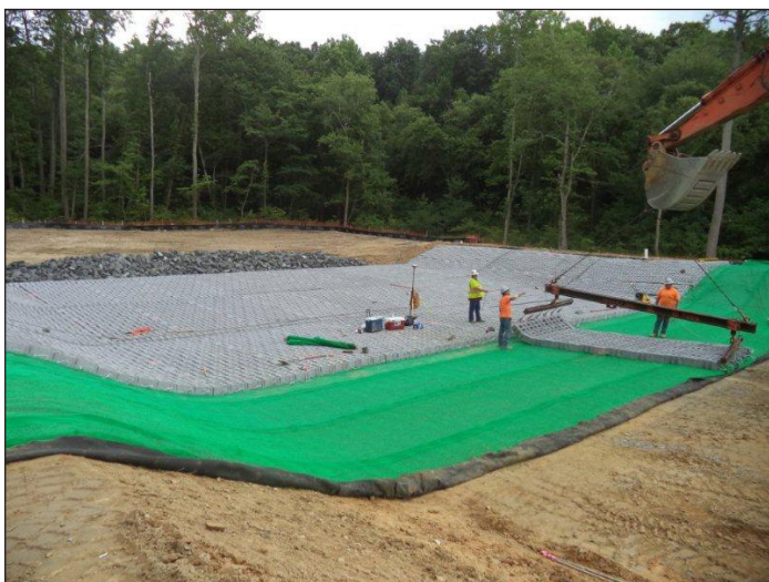
These articulated concrete blocks installed during construction are no longer visible to residents who walk the trails near the dam site.
