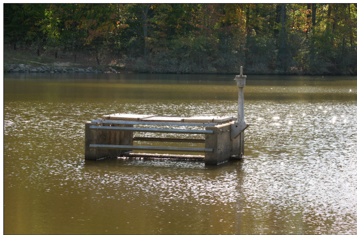
The open spillway riser (above) was replaced to improve public safety and prevent clogging from floating debris.
