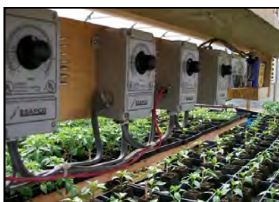
Figure 5. Thermostats mounted in a greenhouse control ventilation by opening and closing vents and controlling fans
