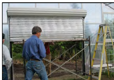
Figure 9. Another way to vent a high tunnel is to install a large door in the end wall. This one is an insulated roll up door
