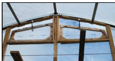
Figure 7. Vents mounted at top of end wall with solar power
