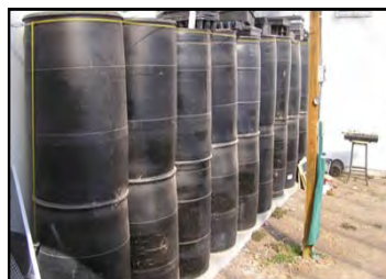
Figure 24. A passive heating system that uses black barrels and water
