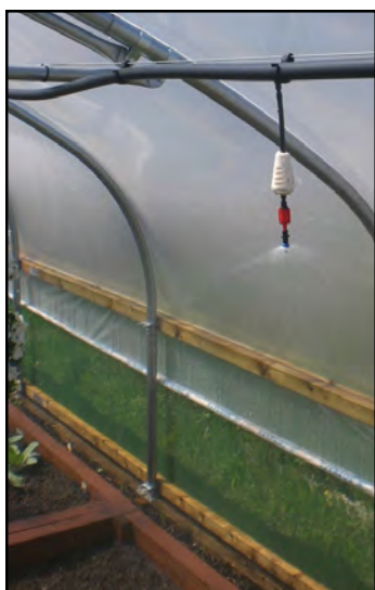
Figure 13. Overhead sprinkler in a high tunnel
