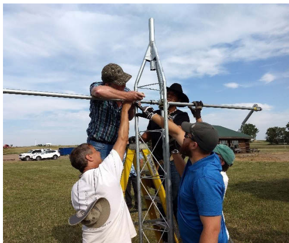
A cross arm supporting the anemometer and solar radiation sensor is installed.
