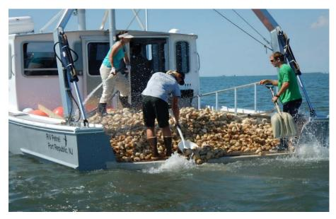
Figure 1.—Spreading cultch on the site selected for oyster reef establishment.
