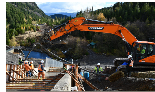
Clear Branch Dam Restoration
