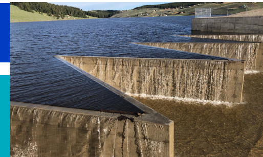
Dull Knife Dam Spillway
