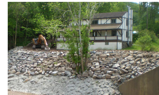
Montour County Stream Bank Restoration
