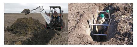
Left image—A backhoe excavation providing a large view of the soil profile and improving access for description and sampling. Right image—Shoring, exit ramps, and other safety measures must be used to protect staff in deep trenches. (Photos courtesy of Wayne Gabriel)
